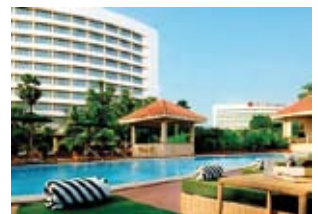
Lakeside Chalet, Mumbai - Marriott Executive Apartment 2 x 1250 kVA, 2 x 750 kVA
